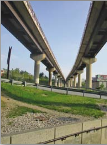
Metrorail near Rhode Island Avenue
